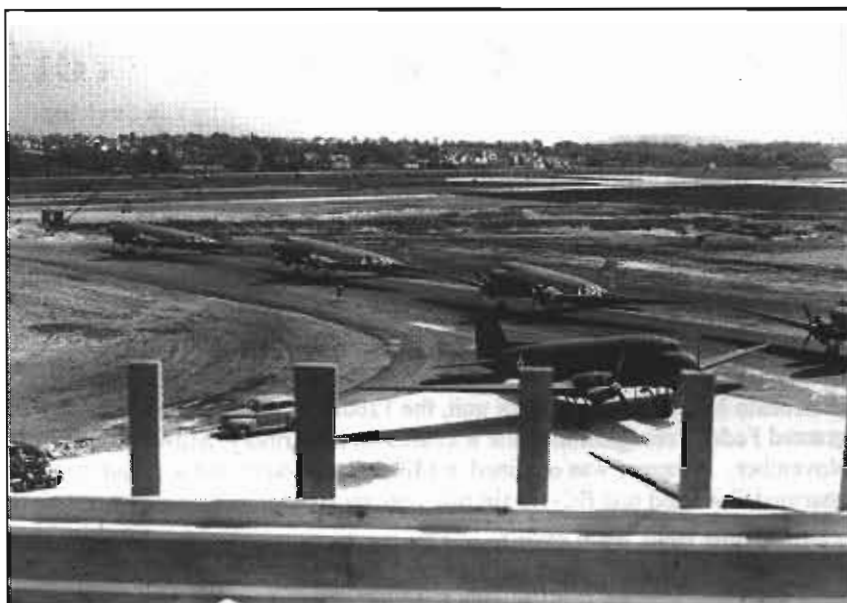
View from atop the newly constructed National Guard hangar showing some of the Douglas C-53 transports used for training troop carrier pilots at Billy Mitchell Field, 1942.
