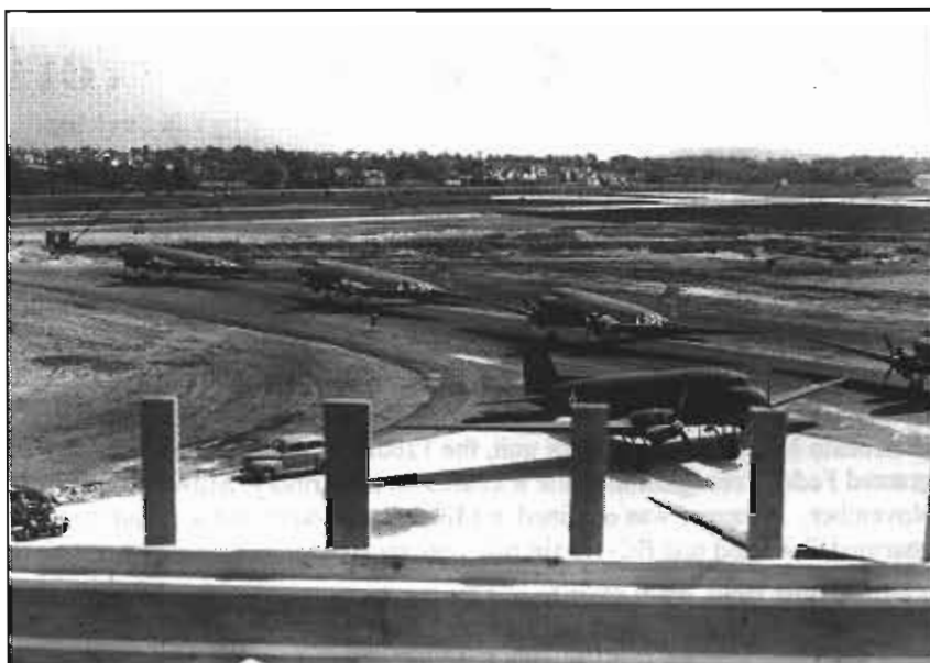
View from atop the newly constructed National Guard hangar showing some of the Douglas C-53 transports used for training troop carrier pilots at Billy Mitchell Field, 1942.
